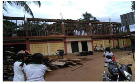
Construction of the new Girls' Hostel
