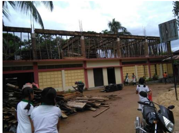
Construction of Bishakha Bhavan (Girls' section)
