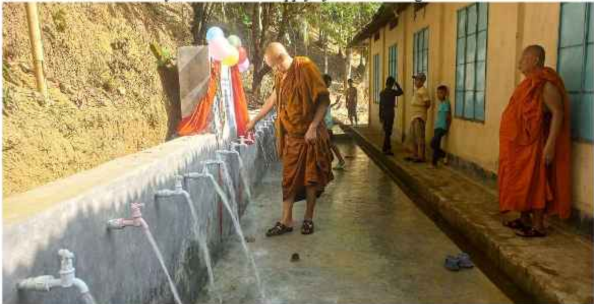
Refurbished Water Supply System at Moanoghar
