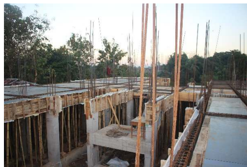
Moanoghar Vocational Trade School building under construction
